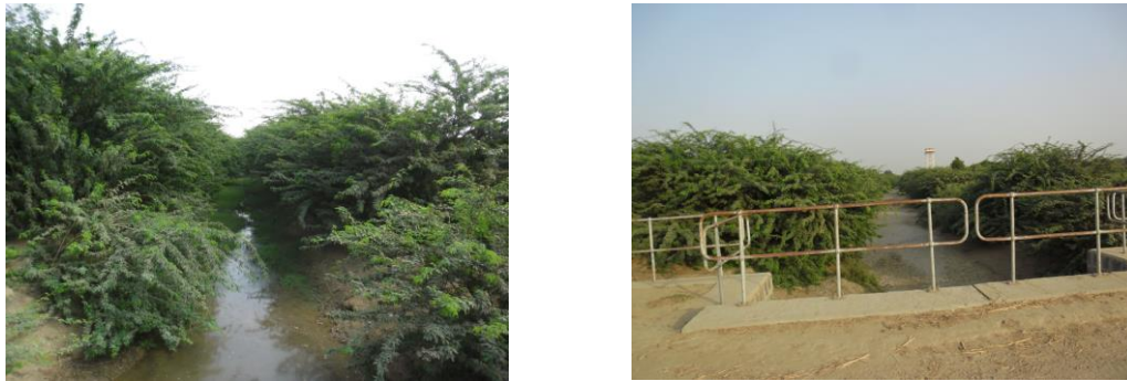
Figure 1: Mesquite Shrub Prosopis juliflora encroaches on canal beds – blocking them and causing drainage patterns to uncontrollably shift.
